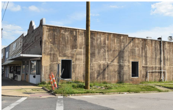
An area of Downtown that requires maintenance.
