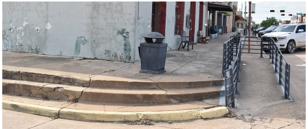
A portion of Downtown Rockdale that could benefit from TIRZ funds for sidewalk maintenance.
