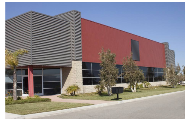
Flex Industrial / R&D Building
