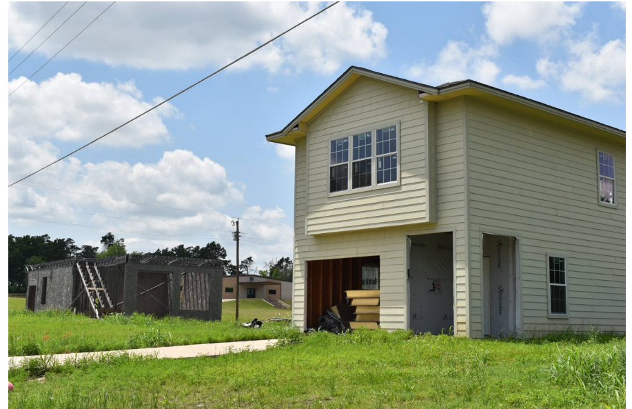
Unfinished housing construction in Rockdale.
