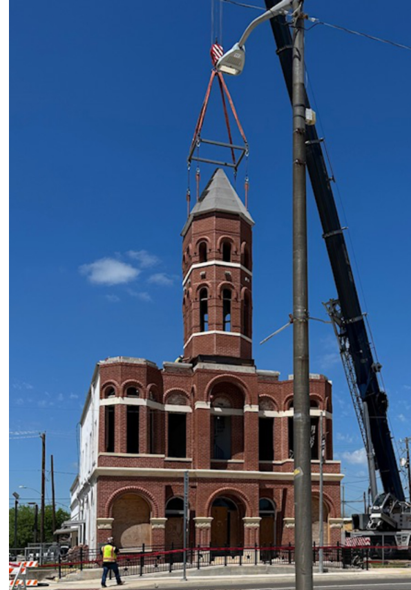
Restoration of the historic 1895 City Hall bell tower
